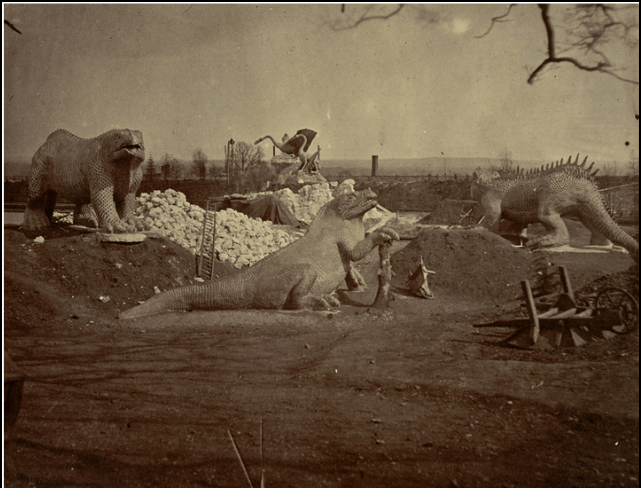
'Models of Extinct Animals', 1855 by Philip Henry Delamotte. Photographic print showing the dinosaurs in construction. Delamotte was commissioned to document the re-erection of the Crystal Palace at Sydenham as well as the installation of the Dinosaurs and their habitat in the surrounding park. Note that the sculptures were constructed on their platforms before the lake was dug and flooded, and before any vegetation was planted
