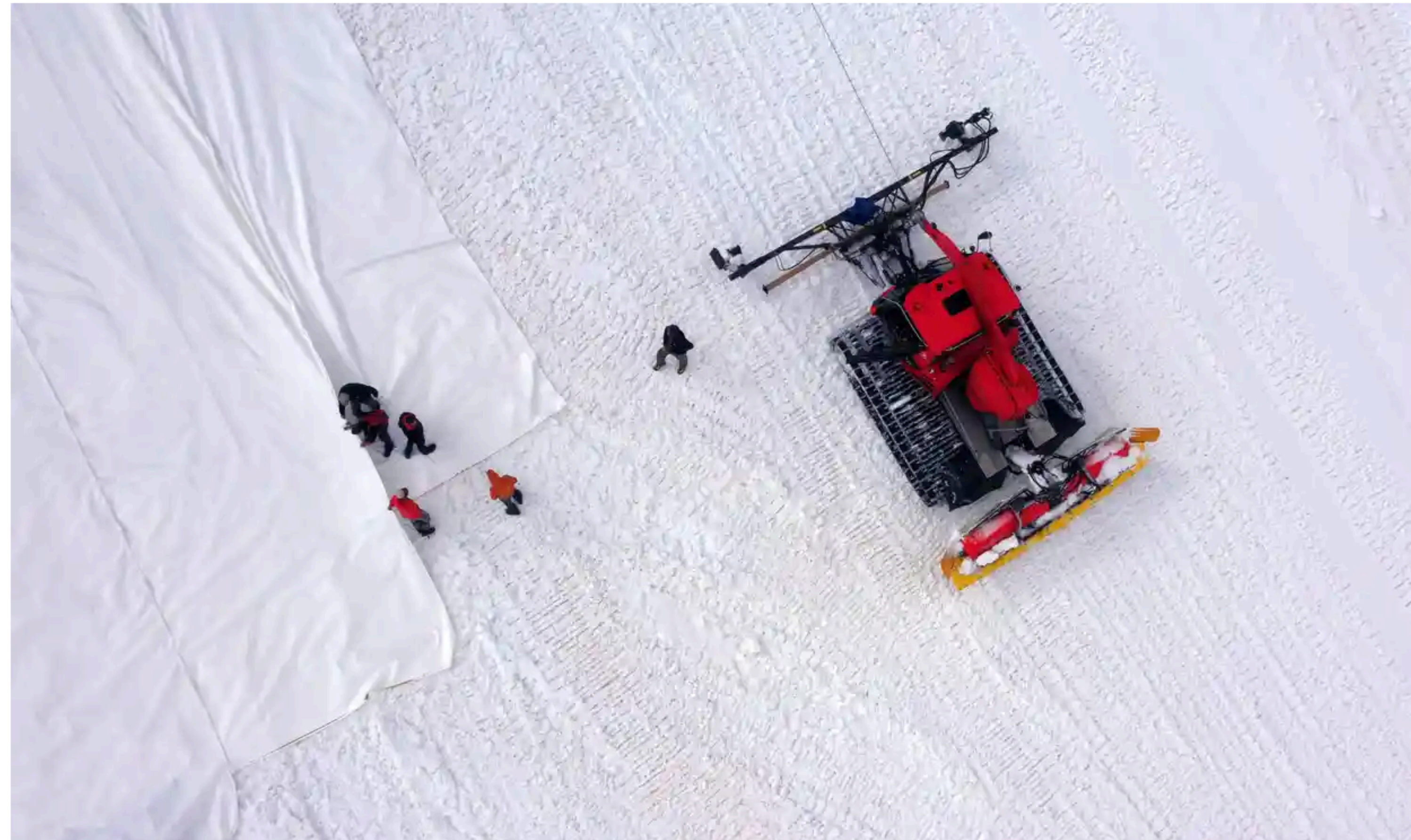
📷 Workers lay out huge geotextile sheets on the Presena glacier in northern Italy. Photograph: Miguel Medina/AFP/Getty Images
