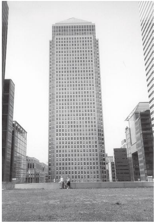
FIGURE 13. A living roof on top of a fifty-story building at Canary Wharf in Central London. Photograph by the author.
