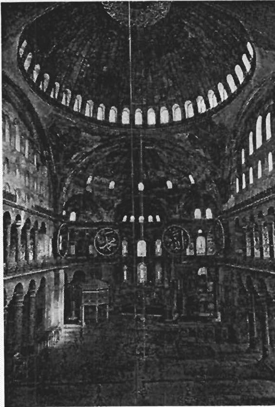
Fig. 4.8 Constantinople (Istanbul), Hagia Sophia, interior looking east. The great dome, over 100 feet in diameter, rises 180 feet above the floor. The interior surfaces are revetted with precious marbles, laid in book-matched panels, and the vaults were originally covered with over four acres of gold mosaic. With light streaming in from the numerous windows, the shimmering surfaces created a magical, ethereal impression. As the sixth-century writer Prokopios suggested, the church could be understood as the dwelling place of the divinity. (courtesy Dumbarton Oaks)
