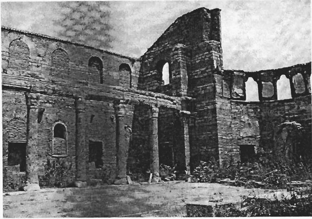
Fig. 4.5 Constantinople (Istanbul), Saint John in the Studios monastery, interior looking northeast. Now in ruins, this is the oldest surviving church in Constantinople, originally built in the middle of the fifth century. A gallery ran above the verde antico (green marble) columns of the side aisles; the supporting brackets can still be seen in the outer wall. (courtesy Dumbarton Oaks)
