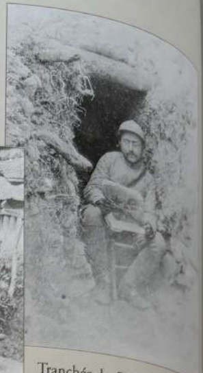
Tranchée du C. devant mon trou. C. trench, in front of my hole.
